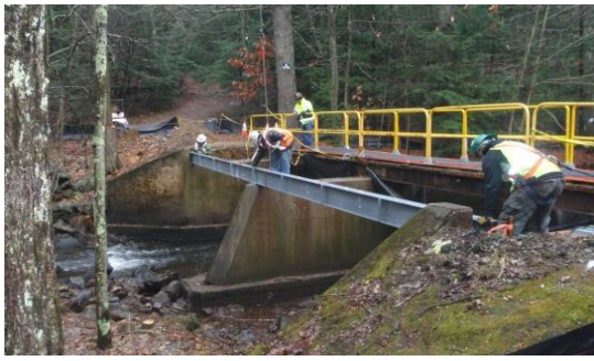
Patterndam Bridge Rehab / Repairs
