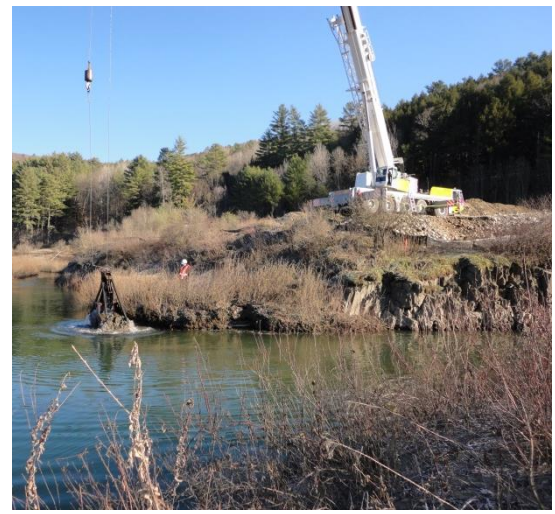
Union Village Dam Maintenance Dredging /Sediment Removal
