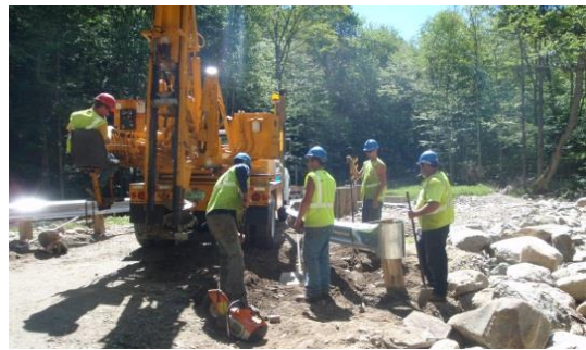
Chittenden Brook | Road Reconstruction
