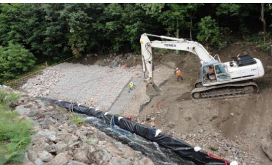
Peters River | Erosion Repairs
