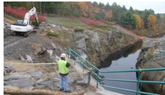
Birch Hill Dam | Stabilization
