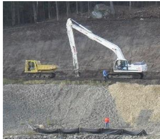
MacDowell Dam | Slope Stabilization
