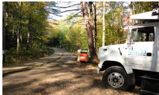
Otter Brook Lake | Access Road Repairs
